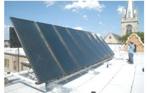
The five systems range from 8 to 16 Solar Panels per building with 360 or 480 gallons of hot water storage. The combined systems include 50 Solar Collectors and are designed to heat over 3,400 gallons of hot water each day or over 900,000 gallons each year.
