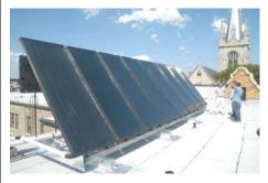
The five systems range from 8 to 16 Solar Panels per building with 360 or 480 gallons of hot water storage. The combined systems include 50 Solar Collectors and are designed to heat over 3,400 gallons of hot water each day or over 900,000 gallons each year.
